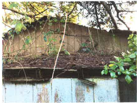
Garage roof collapsed, back of garage collapsed, accumulation of weeds and garbage EXTREME FIRE HAZARD
