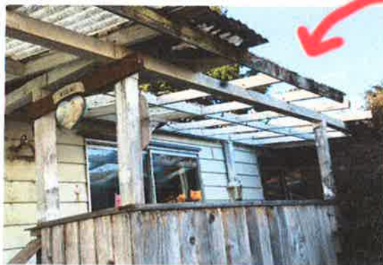
Missing Roofing, Rotten Framing
