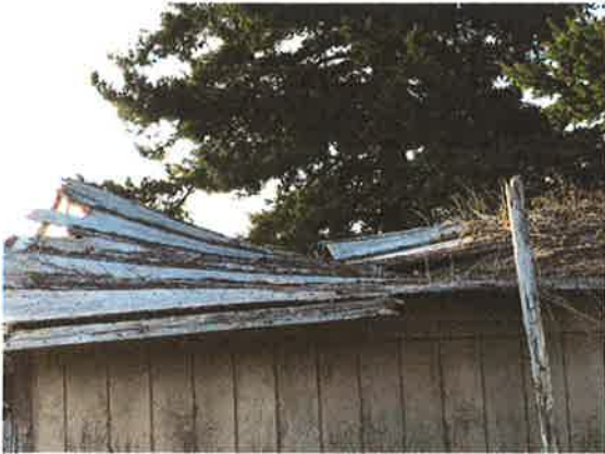
Garage roof collapsed, back of garage collapsed, accumulation of weeds and garbage EXTREME FIRE HAZARD
