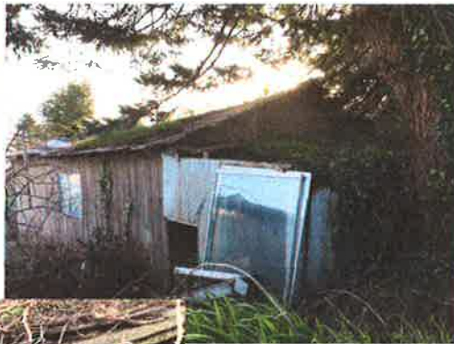
Garage roof collapsed, back of garage collapsed, accumulation of weeds and garbage EXTREME FIRE HAZARD
