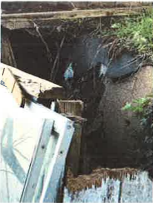
Garage roof collapsed, back of garage collapsed, accumulation of weeds and garbage EXTREME FIRE HAZARD
